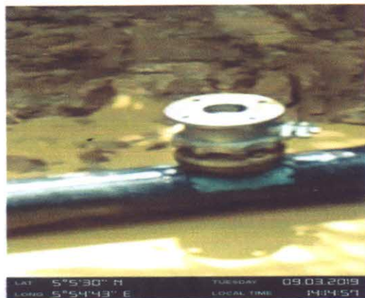
INSTALLED VALVED ON LINE
